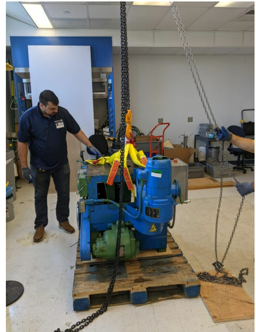
Beam and clamp hoist
